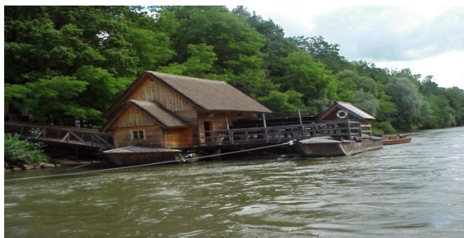
Ship mill on the river Mur
