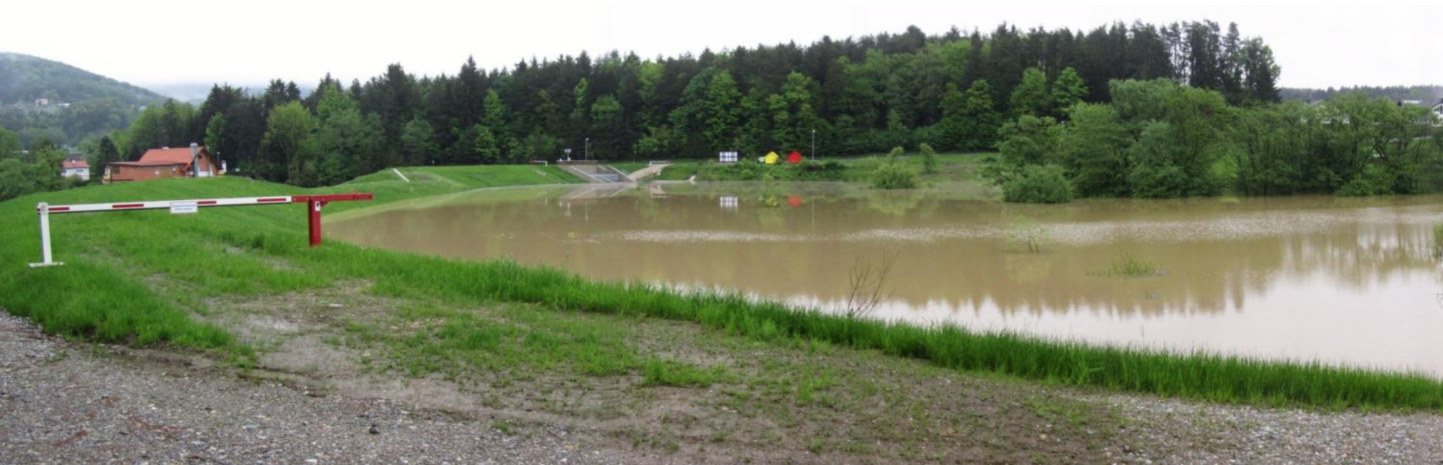
Retention basin Schöckelbach, Graz, 7th June 2013
