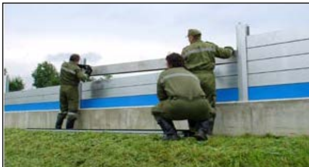
Mobile flood protection
