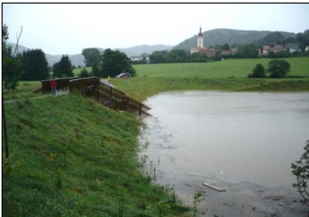
Flood retention basin Gabriachbach, Graz Source: www.wasser.graz.at
