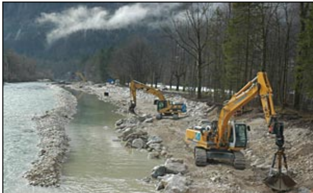
Ecological flood protection, Bad Ischl Source: WWF, Feichtinger
