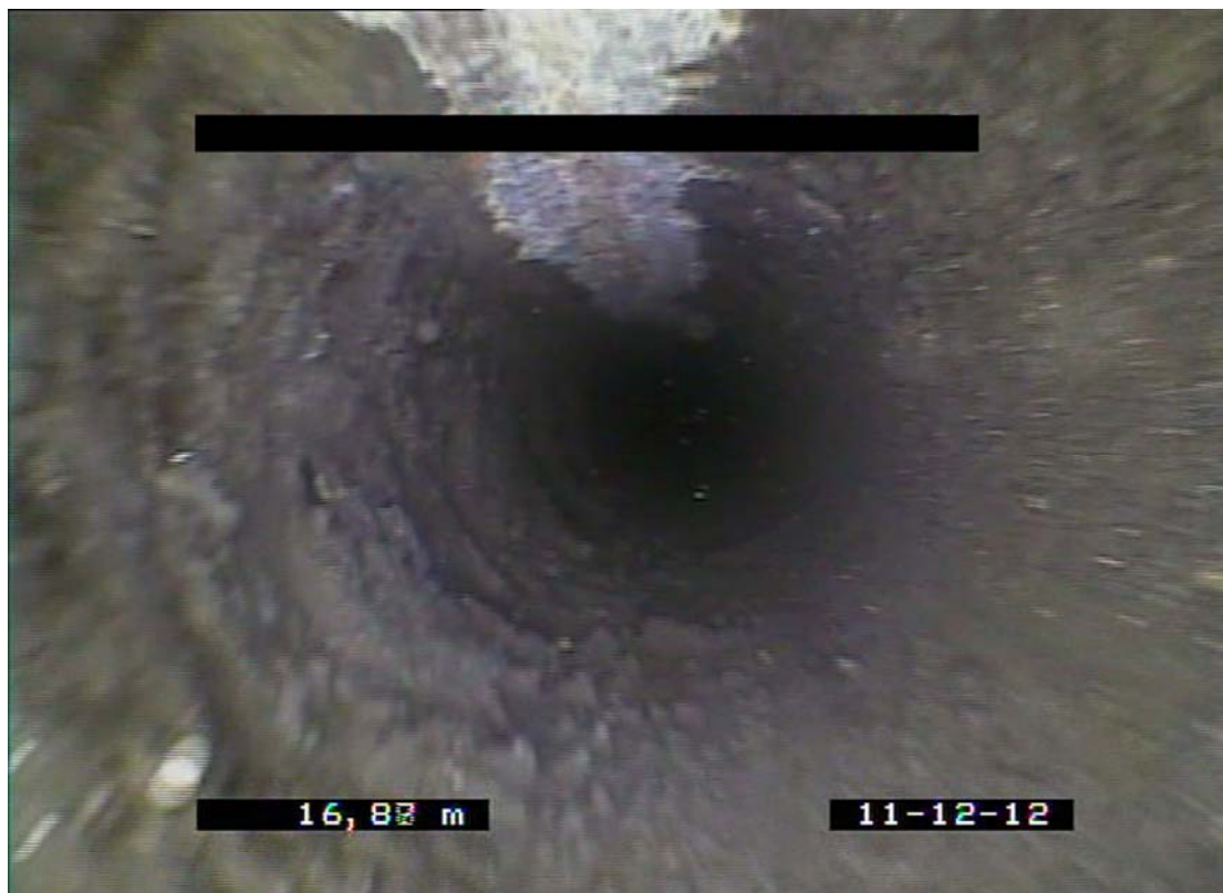
Abb. 25: Starker Rohrbelag
